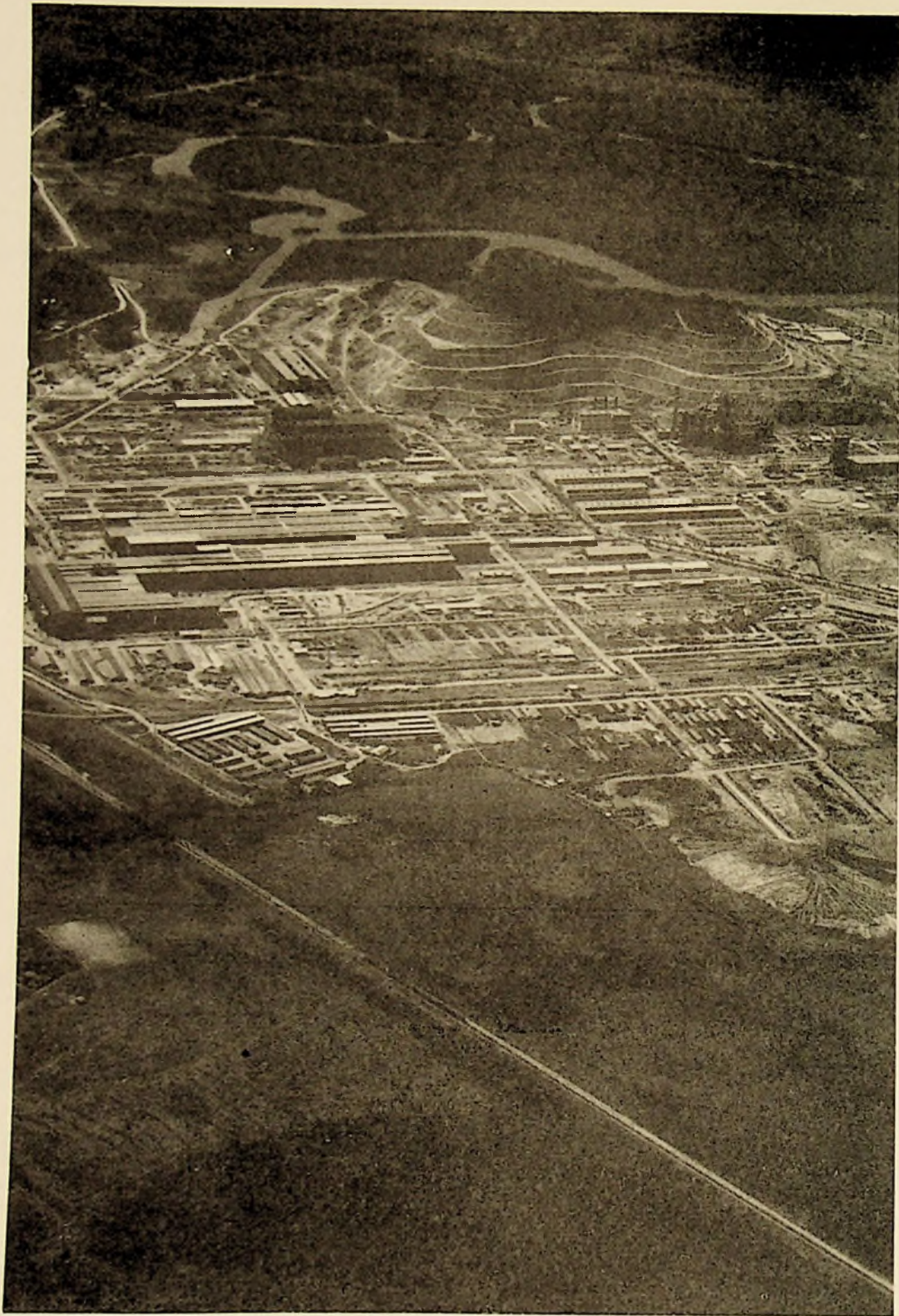
IN SETTING UP ITS STEEL MILL PLANT AT PIAÇAGUERA (SÃO PAULO), THE COMPANHIA SIDERÚRGICA PAULISTA — COSIPA RELIED MAINLY ON BNDE FINANCIAL AID. IT IS EXPECTED THAT THE PRESENT CAPACITY OF 500,000 TONS OF INGOTS WILL BE INCREASED TO 2,000,000 TONS IN ITS FINAL STAGE.
